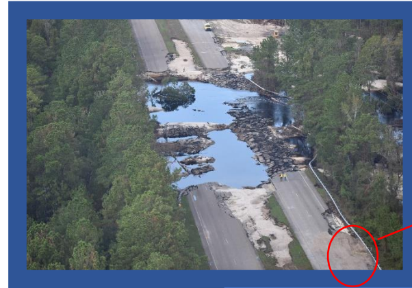
Raw water main washout location
